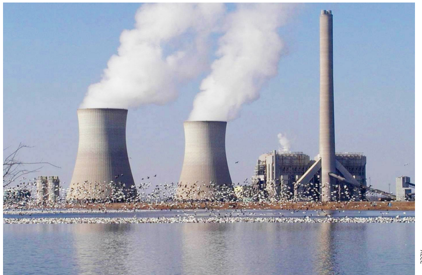
Independence Steam Electric Station will cease operation in 2030.
