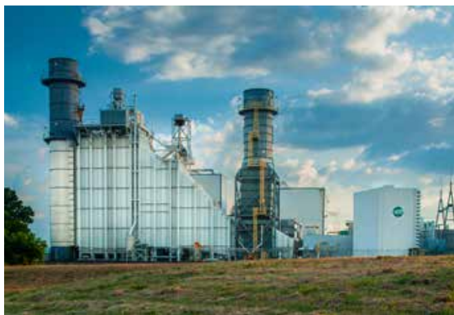
AECC's Thomas B. Fitzhugh Generating Station, a natural gas plant in Ozark, can produce 170 megawatts (MW).
